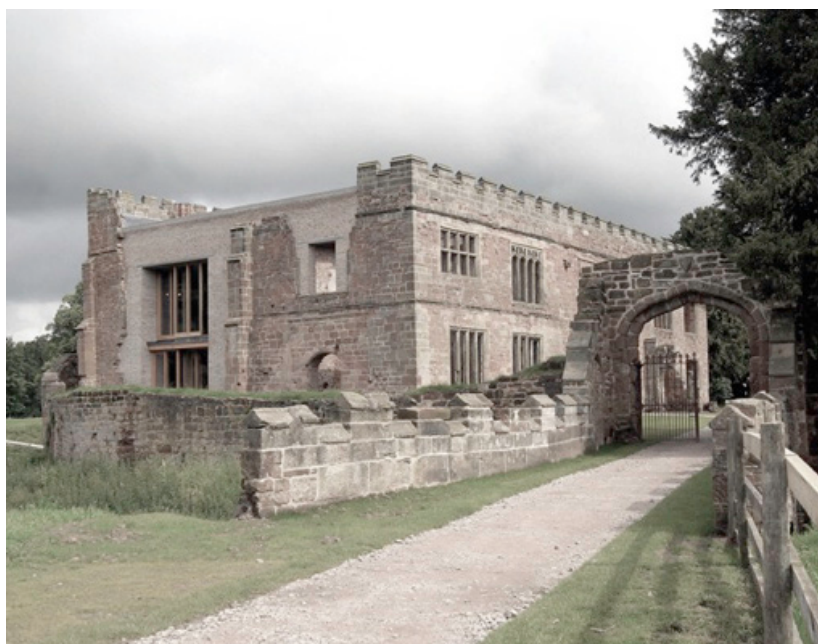
Fig. 24. Astley Castle , Witherford Watson Mann Architects, 2012, Engeland (Enpundit, n.d.)
